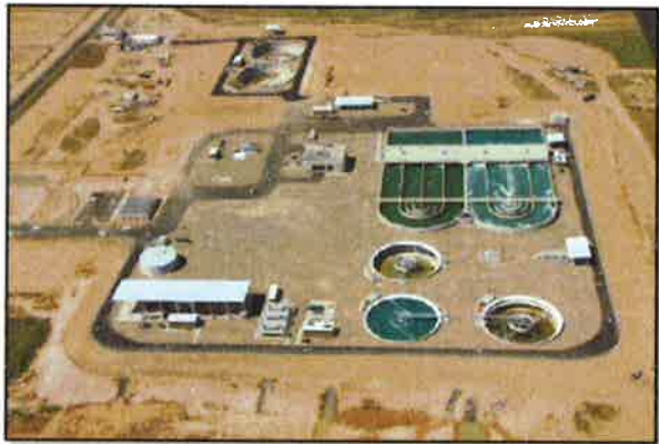
WWTP at 530 South Bert Crane Road
